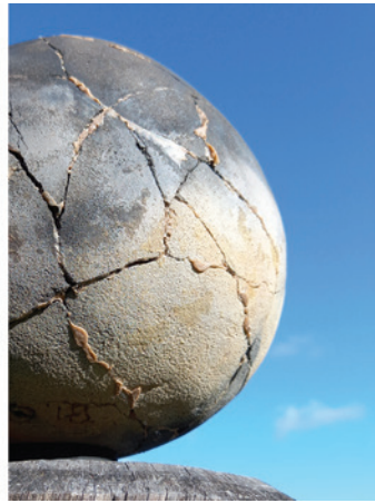
IS-30 HOLDING IT TOGETHER
